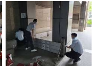
Wan-Da-Tong Access Flood Disaster Education Training - Installation of Flood Control Thresholds (2)
