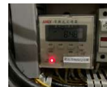
➤ Addition of a time management controller to the spotlight.
