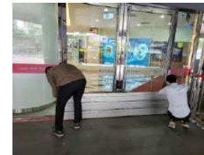
Wan-Da-Tong Access Flood Disaster Education Training - Installation of Flood Control Thresholds (1)
