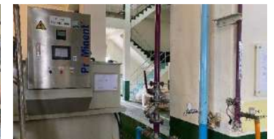
Added reclaimed water piping to sludge chemical treatment systems
