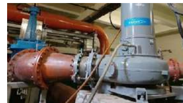
Added reclaimed water piping for pump cooling
