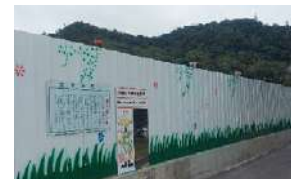
Installation of overflow prevention facilities around the fence
