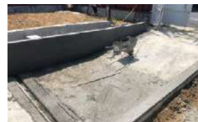
Installation of cleaning equipment and sand sink
